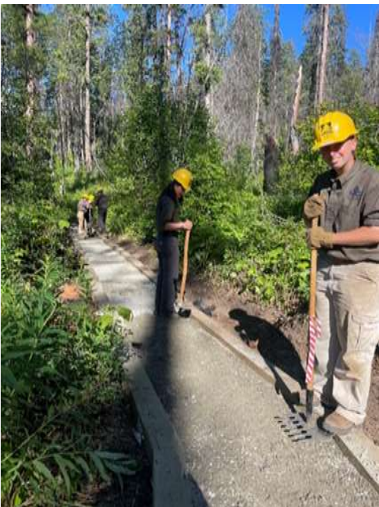
NYC crew members compact a course of gravel.
