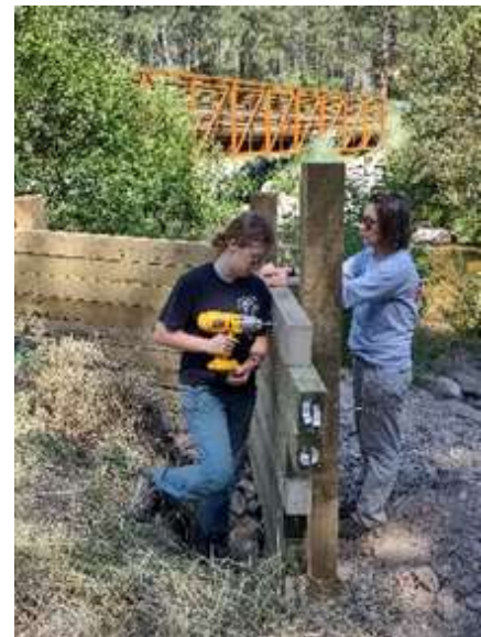
NYC and FS attach horizontal timbers.
