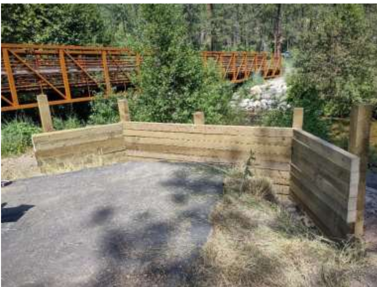
Retaining wall ready for backfill.
