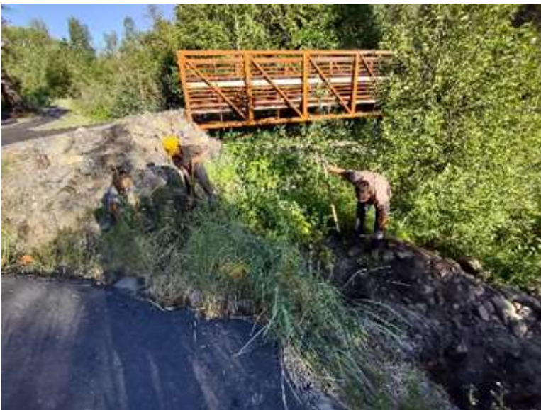
NYC prepping timber support holes
